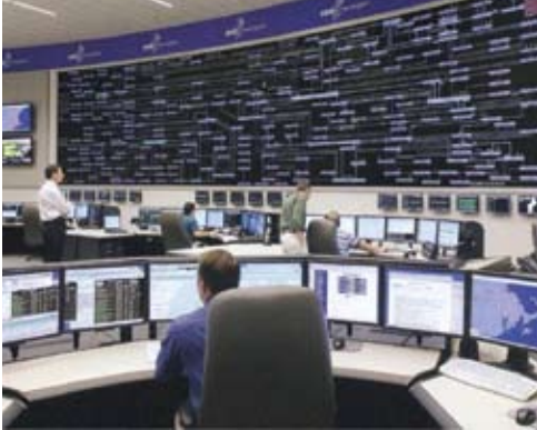
Control room of a transmission system operator
